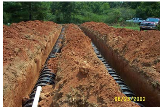
Figure 5. Chamber systems are sturdy plastic molded into a dome shape and the sides are slotted to allow for seepage into the soil.
